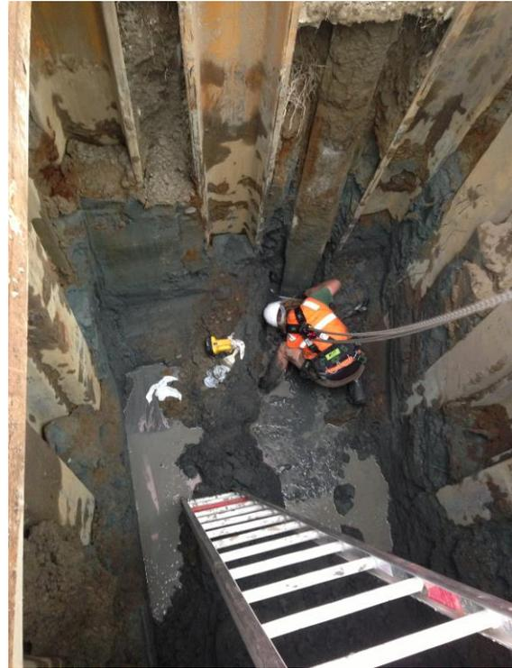
Checking for damage in the upper 4 m of the pile. Our analysis determined that damage, if any, would be found in this part of the pile.
